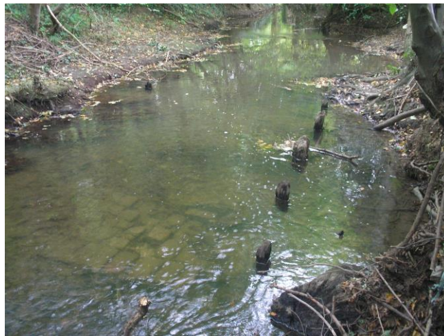
Surviving oak revetment piles and earlier weir near Maidens Bridge
