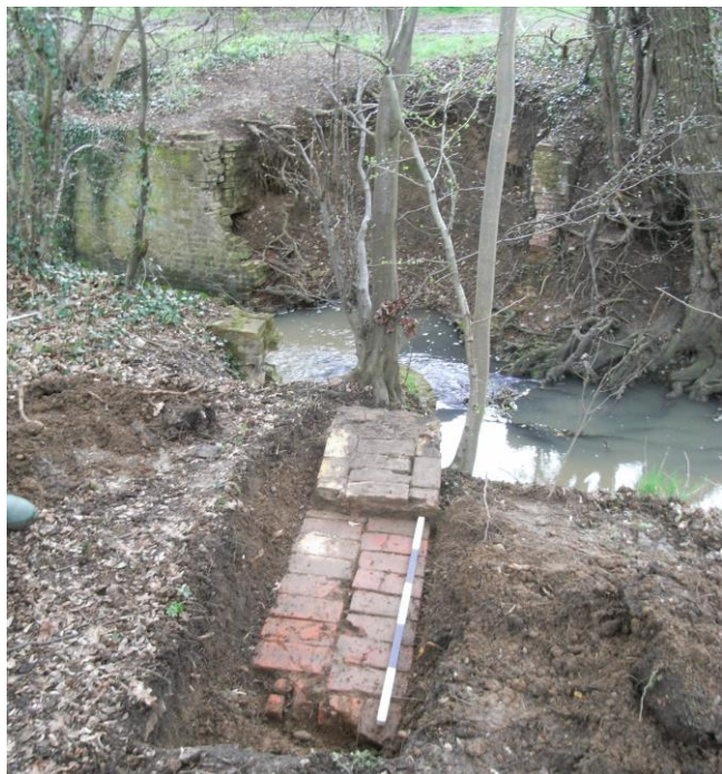
Partially collapsed south bank of the eastern cascade. The two sections of wall on the south bank are those represented above the water-line in section AA on p*. (Ed.)
