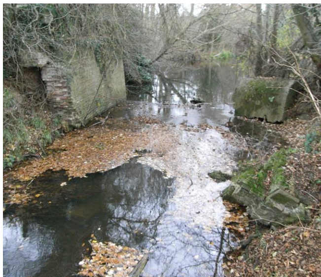
The western cascade, looking downstream from within the second reservoir (Ed.)
